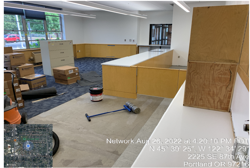
HPMS Admin Office – new ceiling, new lighting, updated paint, new case work, new counters and new flooring
